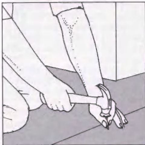
1. Nail along edges about 8" OC, using ring-shank or screw-shank nails.
